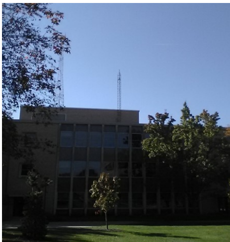
Image: The amateur radio tower on Kettler Hall today. The tower is located in the center of the photo. The main communications tower can be seen in the left background of the photo. The photo was taken in 2023.
